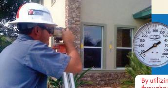
The structure is monitored for movement and the gauge is monitored for high pressures. Once the pressure gauge reaches 300 psi, the grout pipe will be extracted in 5' increments and the process starts over until the soils have been stabilized.
