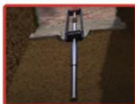
Pier sections are hydraulically driven to the point of refusal.
