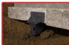
Area prepped with bracket secured against footer, ready for installation.
