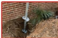
Area prepped with pier next to footer, ready for installation.
