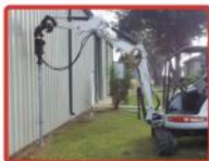
Equipment drives helical piers to the point of refusal.
